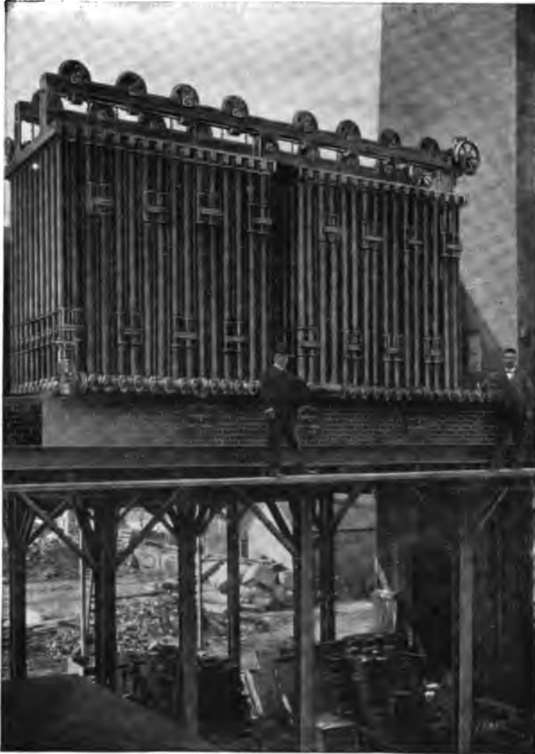
FIG. 46.—Green Fuel Economizer.
